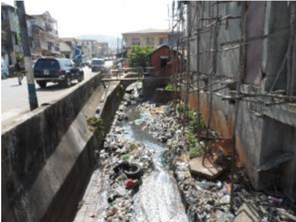
Figure 8: Open drain in central Freetown Source: T. Binns personal collection
