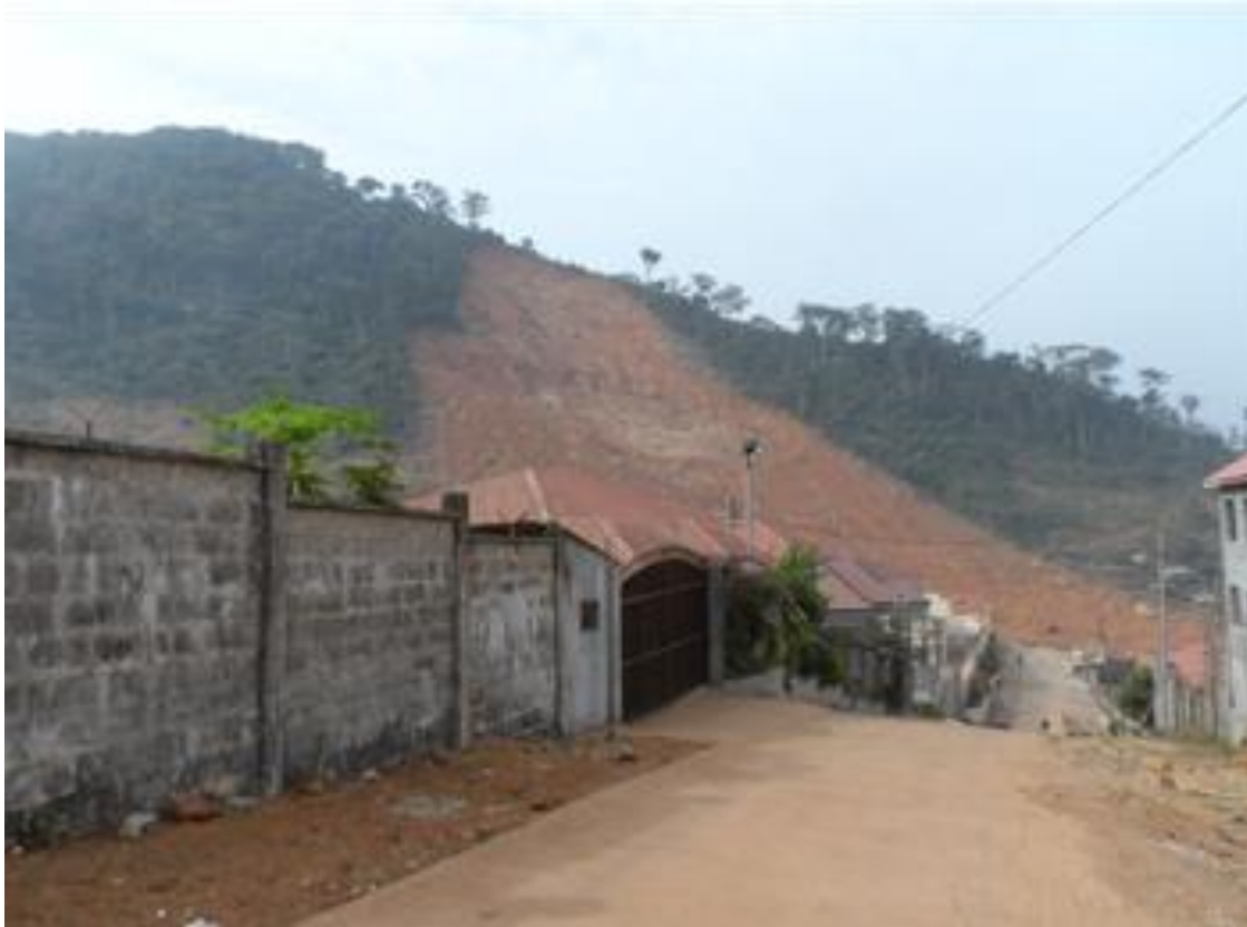
Figure 10: Landslip near Regent, August 2017
