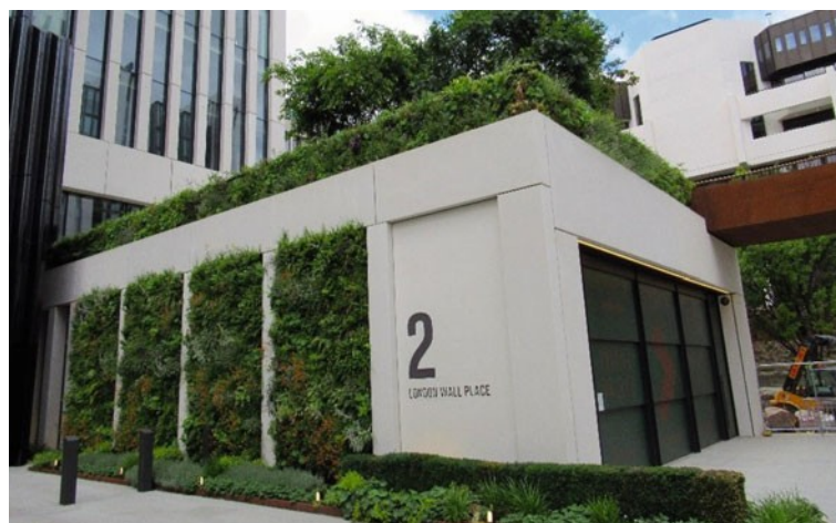
Fig. 10.7 London Wall Place. Photograph taken by A. Russo on June 15, 2018
