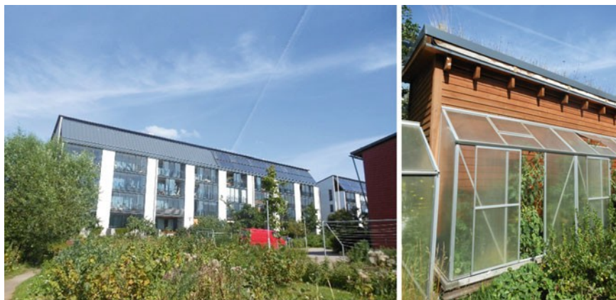
Fig. 10.1 Eco-Viikki, Finland—(left) ecological building and “green fingers” with gardening plots, (right) green roof and greenhouse. Photographs taken by A. Russo on August 15, 2012
