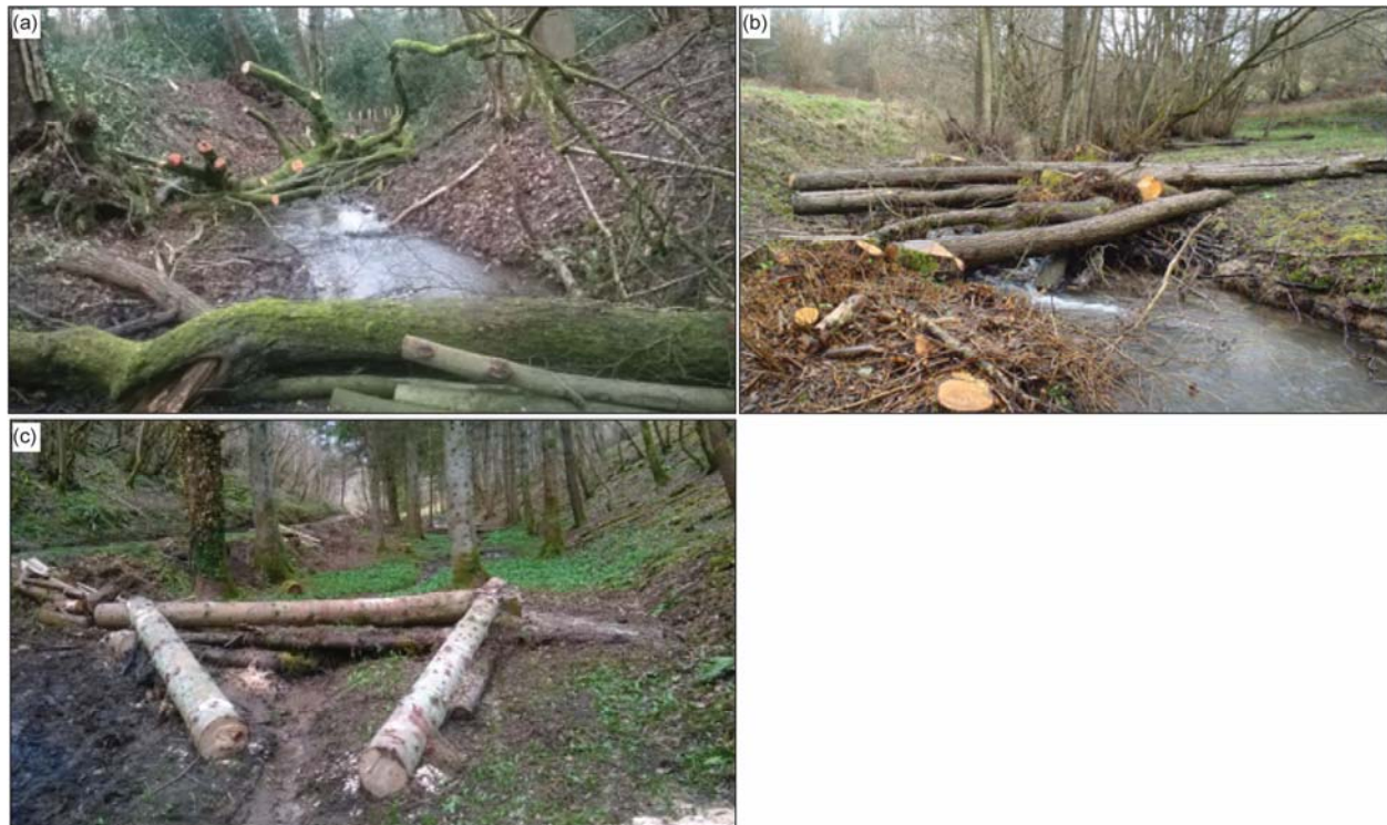
Figure 2: Examples of LWD implemented in the Stroud Frome Catchment: (a) natural, (b) semi-natural design, (c) structured
