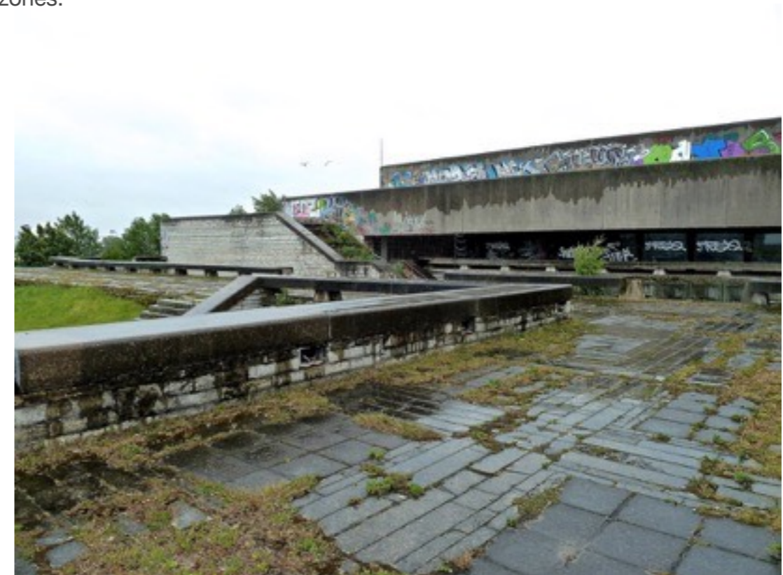
Linnahall Olympic structure in Tallinn, Estonia, built for yachting events of the 1980 Moscow Olympics (Photo © Owain Jones, 2015)
