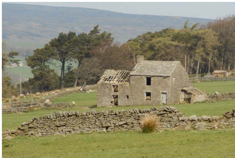
Figure 3.1: Derelict walls and buildings in the enclosed valley landscape
