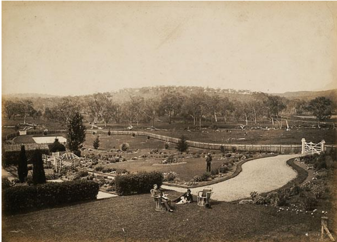
Fig. 1.29 Homestead Garden showing perimeter fence and carriageway
