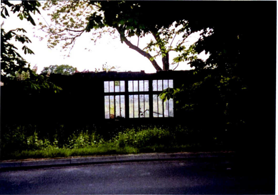
Fig 318 Derelict building Photograph: 6 x 4 in
