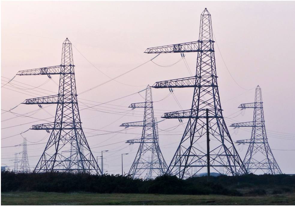
Electricity pylons near to a coal-fired power station
