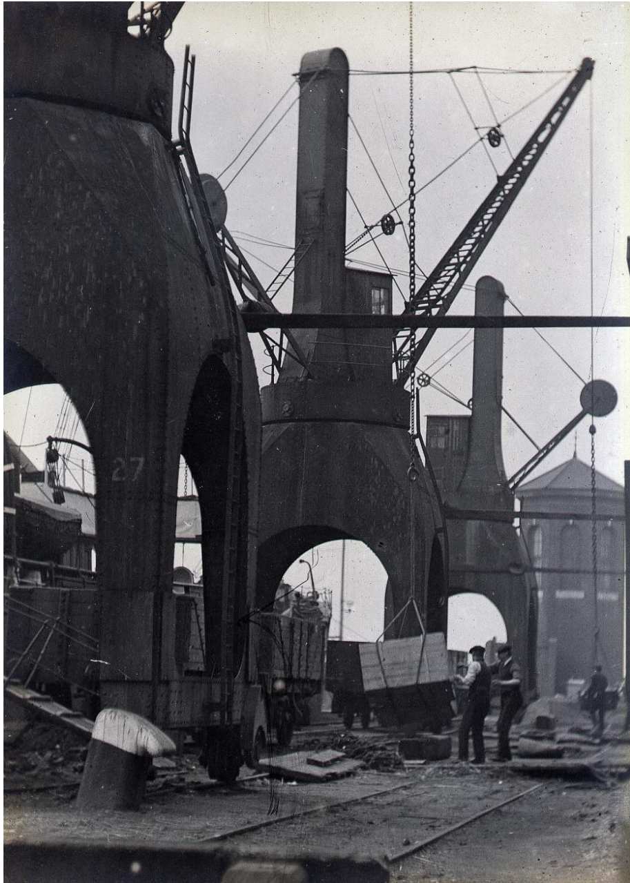
Fig. 8.4 Walter Benington, Tilbury Docks – Cranes, unloading goods “Made in Germany” (1912) Bromide 254 x 182 mm. (photo: © Benington Collections)
