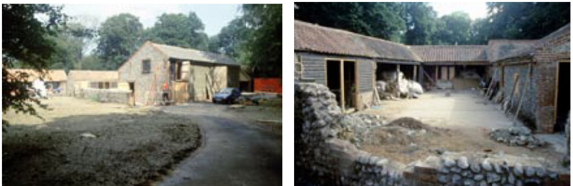
Figure 6.14: Sheringham Park barn undergoing conversion
