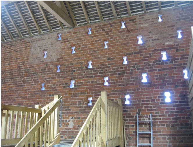
Figure 6.2: Ventilation holes
