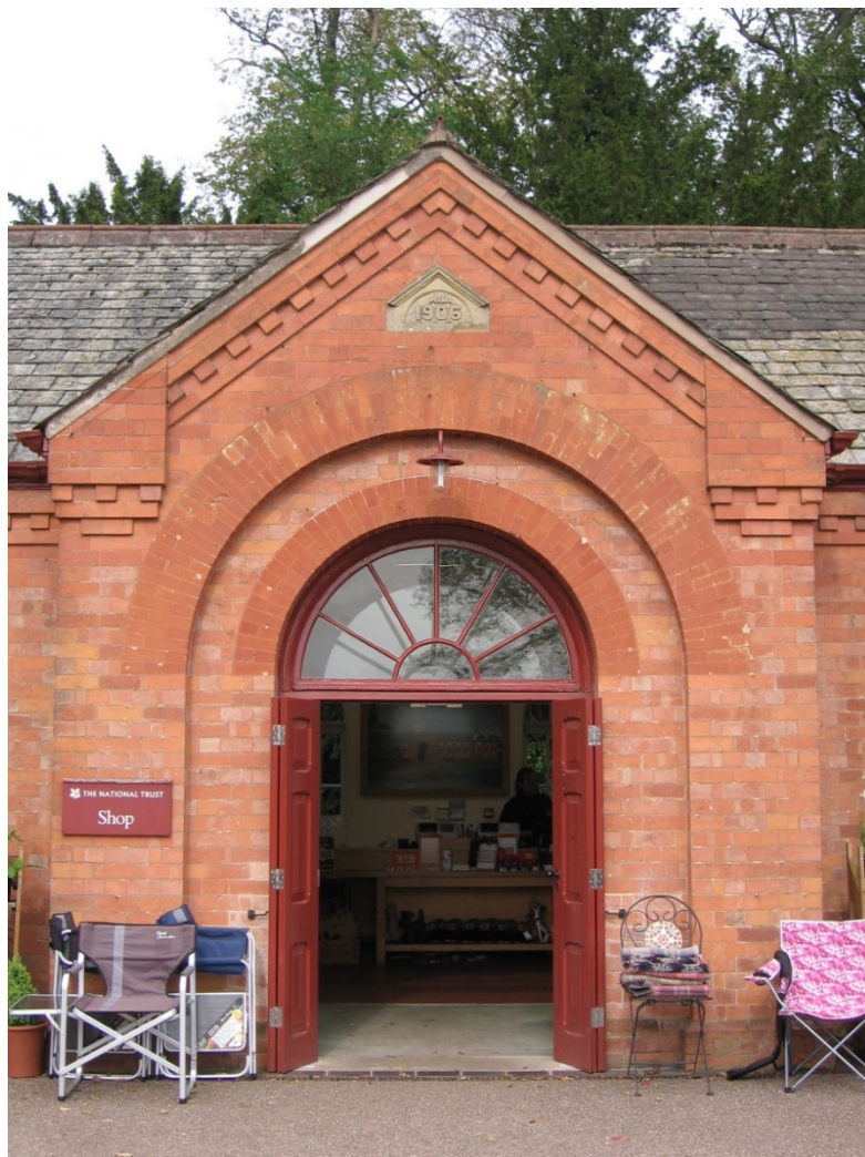
Figure 6.33: Old Laundry Cottages entrance
