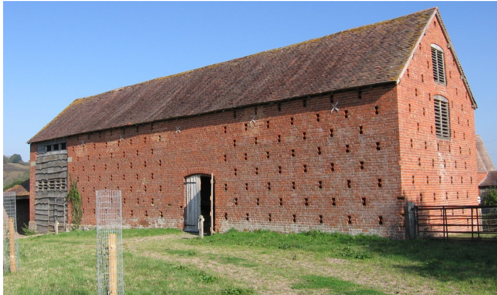
Figure 6.1: Oast House Barn post conversion works
