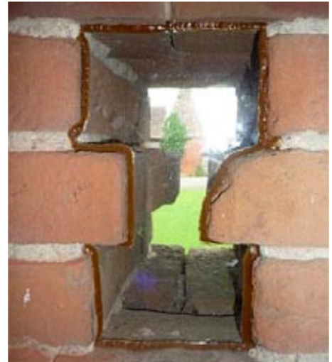
Figure 6.3: Ventilation hole
