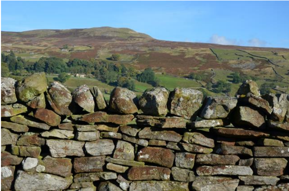
Figure 4.24: Coping stones, Swaledale
