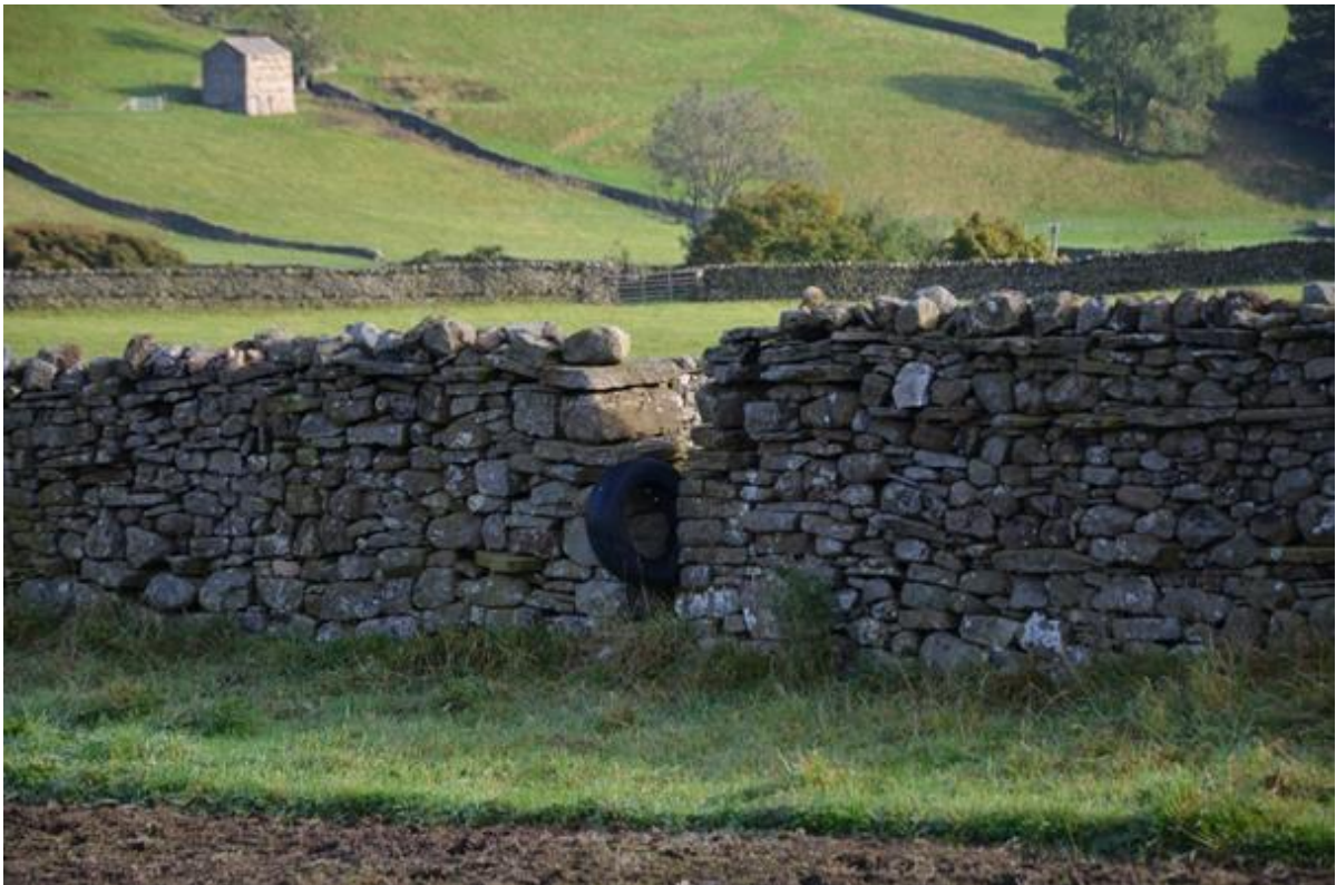
Figure 4.26: Style in a stone wall, Swaledale
