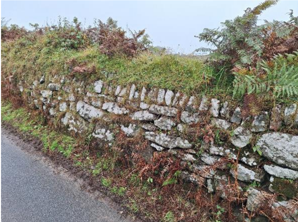
Figure 4.34: Roadside stone-faced bank, Dunstone
