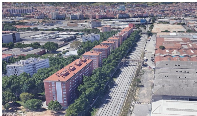
Figure 28. The replacement dwellings at La Verneda in 2020. Compare with Figure 11 .
