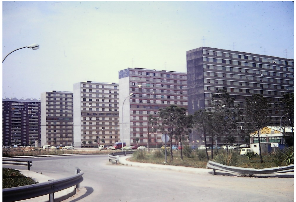
Figure 23. The Bellvitge estate in 1976, planned by the CUB but developed by the private sector. Photo: M. Wynn.
