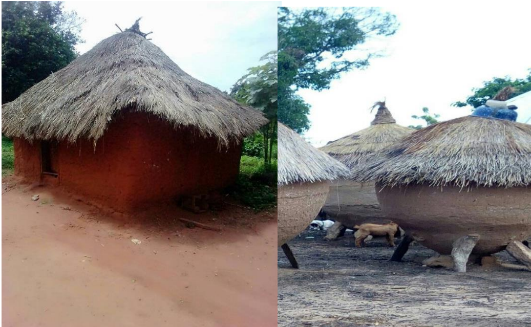
Figure 6.16: Storage type: Mud walls with thatch roofs Credit: Author, from the field.
