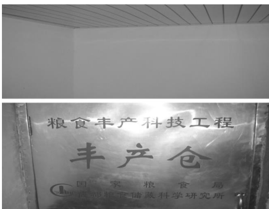
Figure 3.8: Concrete grain storage in China.
