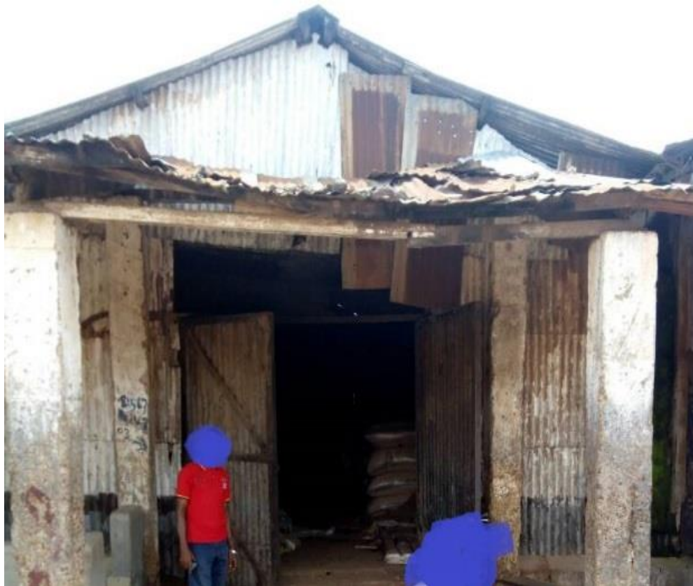
Figure 6.17: Storage type: Plastered mud/concrete walls with zinc roofing sheets Farmers do not live with the grains in this type (non-live-in).
