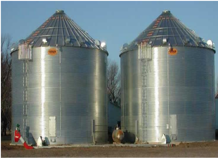
Figure 3.3 - Grain Storage Bins
