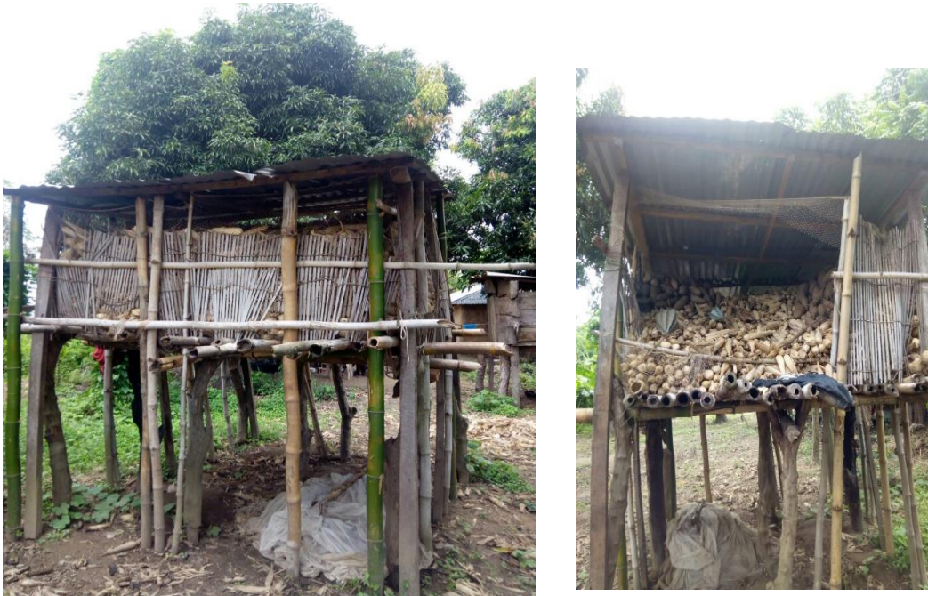
Figure 6.15: Storage type: Thatch walls with zinc roofing sheets. Credit: Author, from the field.
