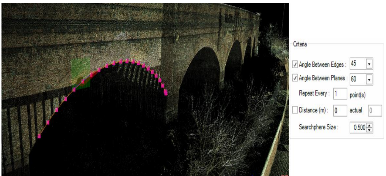
Figure 5.32 Edge Stream detection along a curve of the bridge
