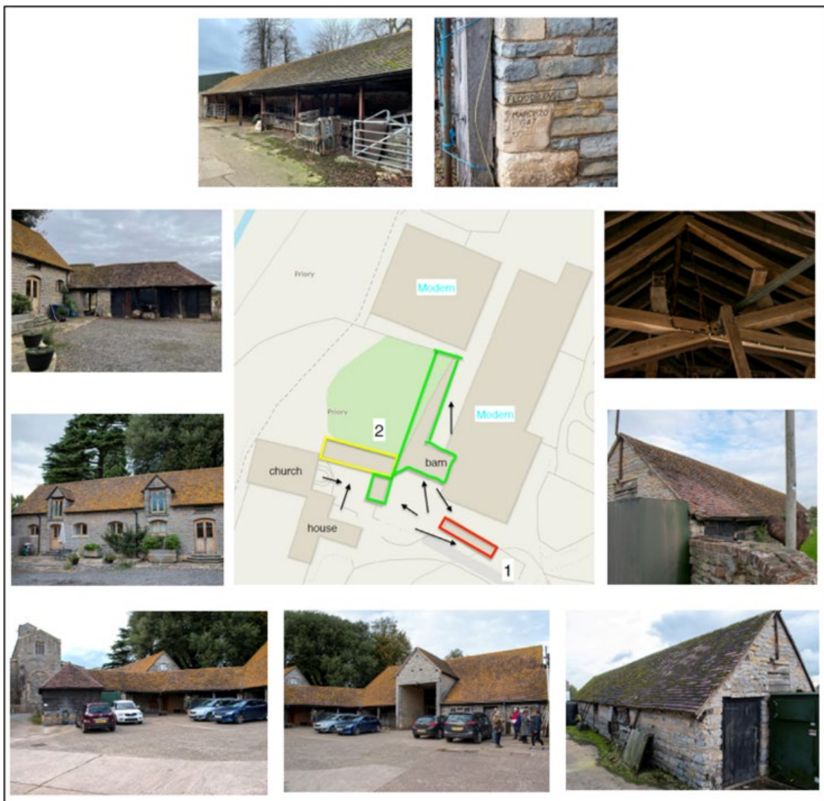
Figure 2.5-5 Example photographs taken for 2 building ranges
