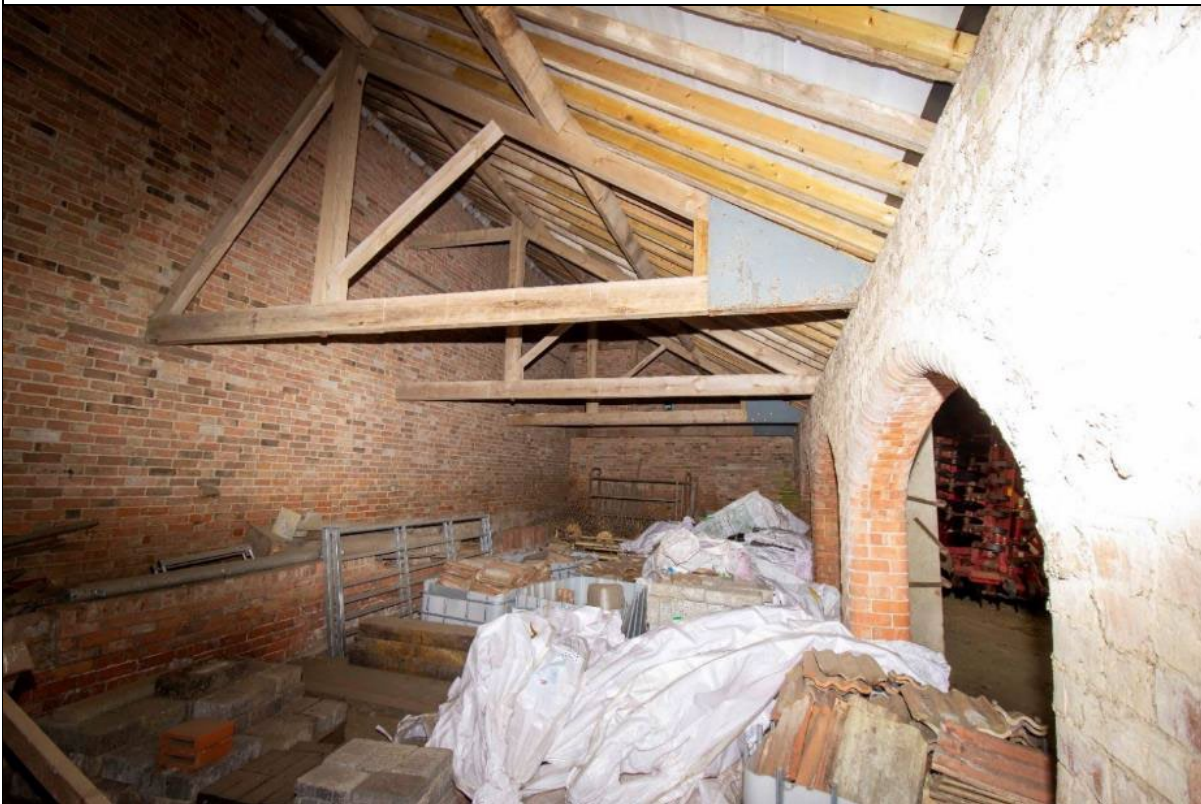
Roof repairs. © Peter Gaskell/CCRI
