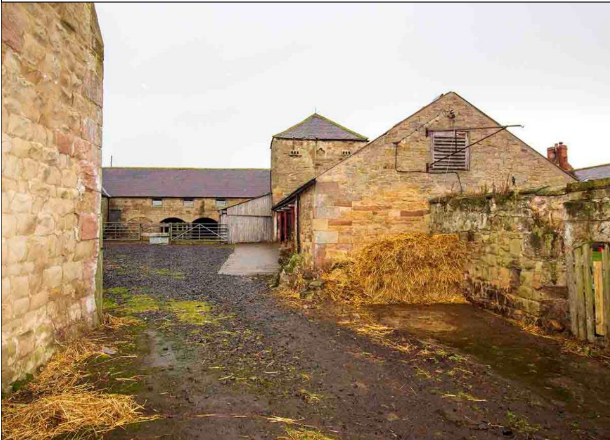
A view into one of the farmyards, showing the fine detail to the masonry and the tall dovecot which was used as a symbol of high status on farmsteads in this area. © Peter Gaskell/CCRI
