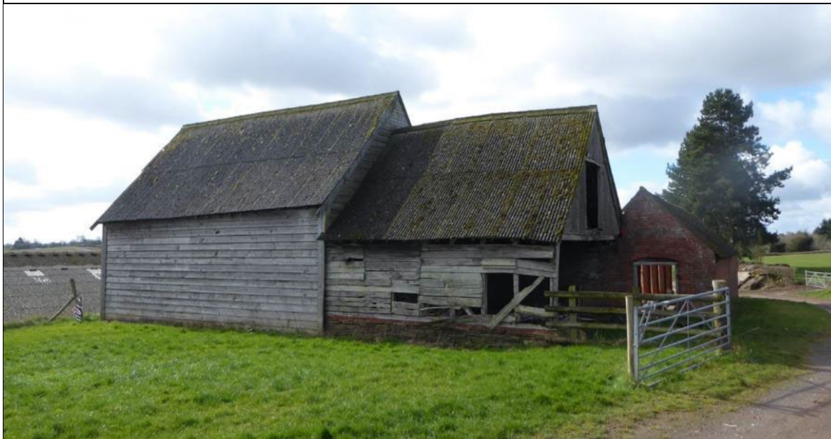
The weatherboarded hay barn and its attached waggon shed. © Jeremy Lake/CCRI
