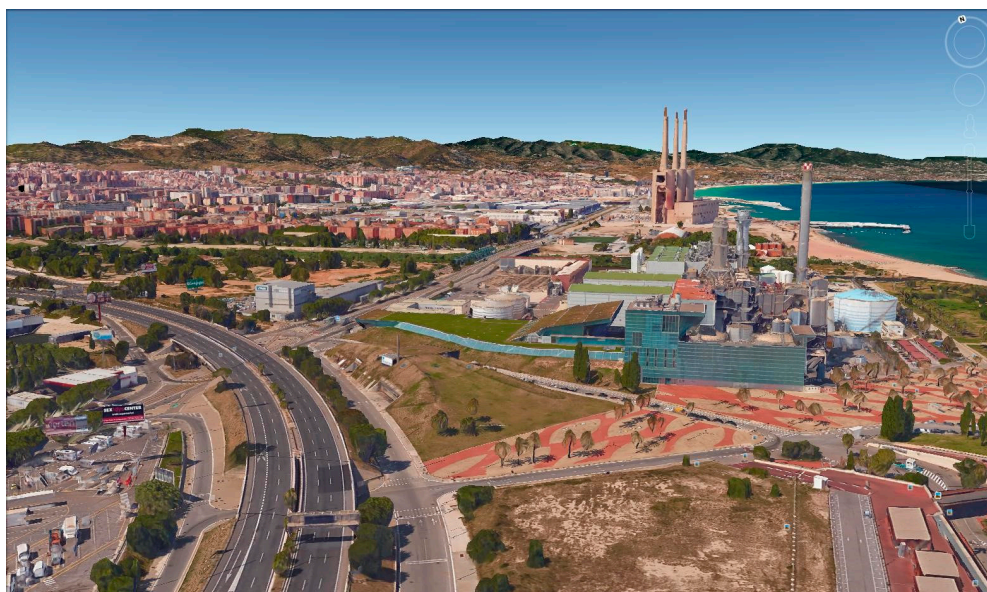
Figure 25. Campo de la Bota in 2019. The new coast road and urban park, with the recycling plant behind (compare with Figure 21) (source: Google Earth).
