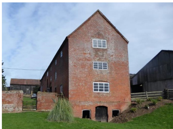
Figure 2: This large brick range on a farm in Herefordshire has a cellar for cider barrels below the cider mill and a kiln for drying hops. © Jeremy Lake/CCRI
