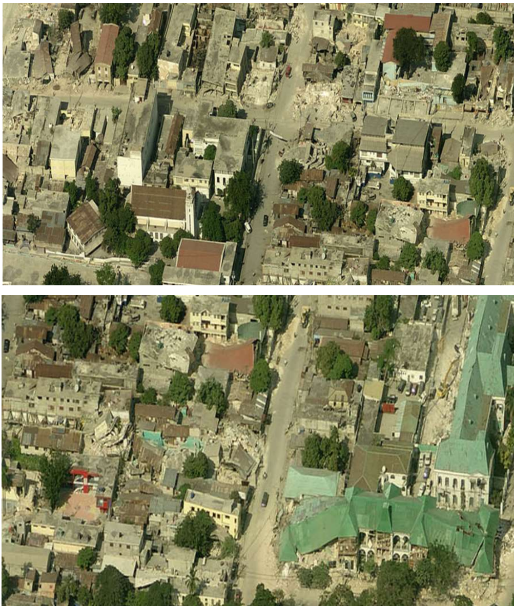
Figure 4.8. Oblique aerial imagery showing roof and façade view of damaged buildings
