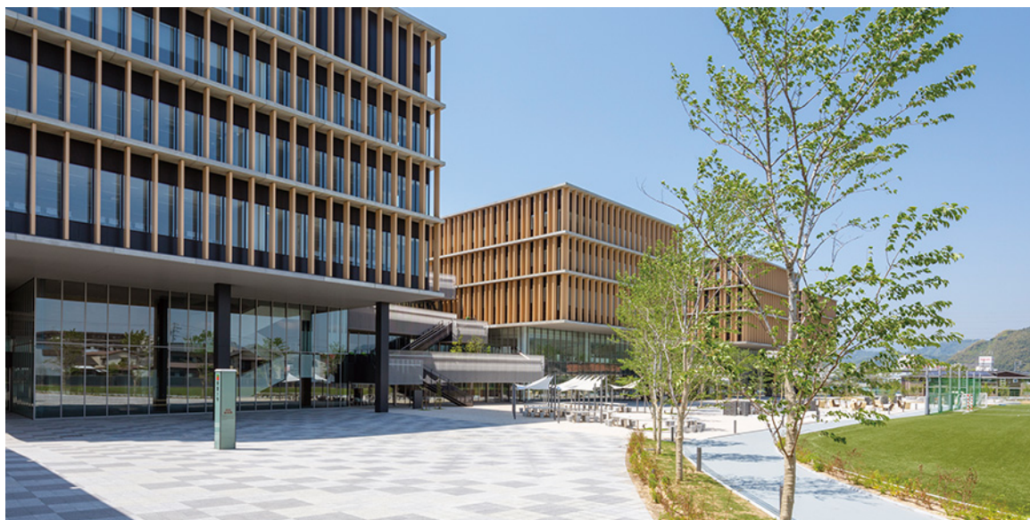
Figure 4: A view of the main buildings at the campus, where this study took place. Click on the image to try a virtual tour. Photo compliments of Tokoha University.
