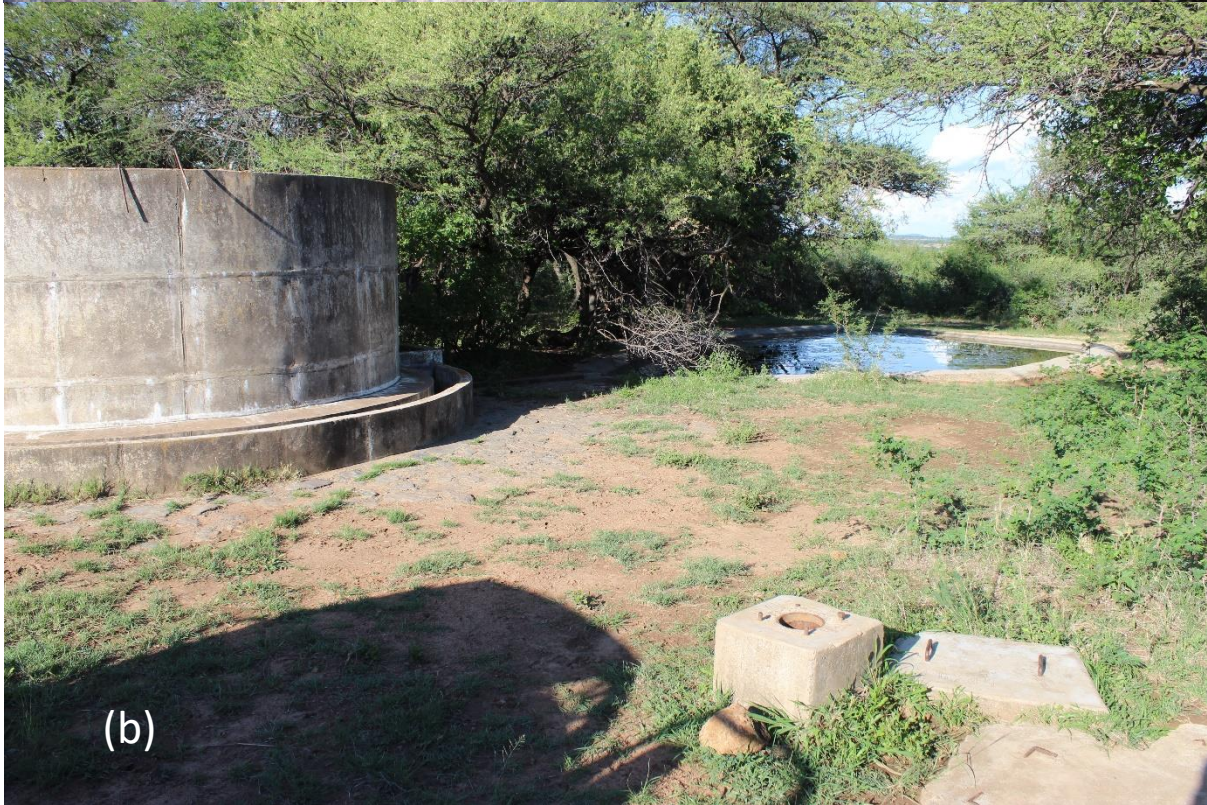
Figure 17: The two different types of pans found at the study site. 10(a) shows a continual flow plan, Marula pan, the pipe at the bottom right of the photo is left on to keep water flowing into the pan, the amount of water flowing can be adjusted dependant on how often the pan is used by animals. 10(b) shows a pumped pan, Kudu pan, these pans are pumped using a bore hole, the concrete structure at the bottom of the photo. These pans are pumped ca. every two weeks in the dry season and once a month in the wet season, dependant on use by animals.
