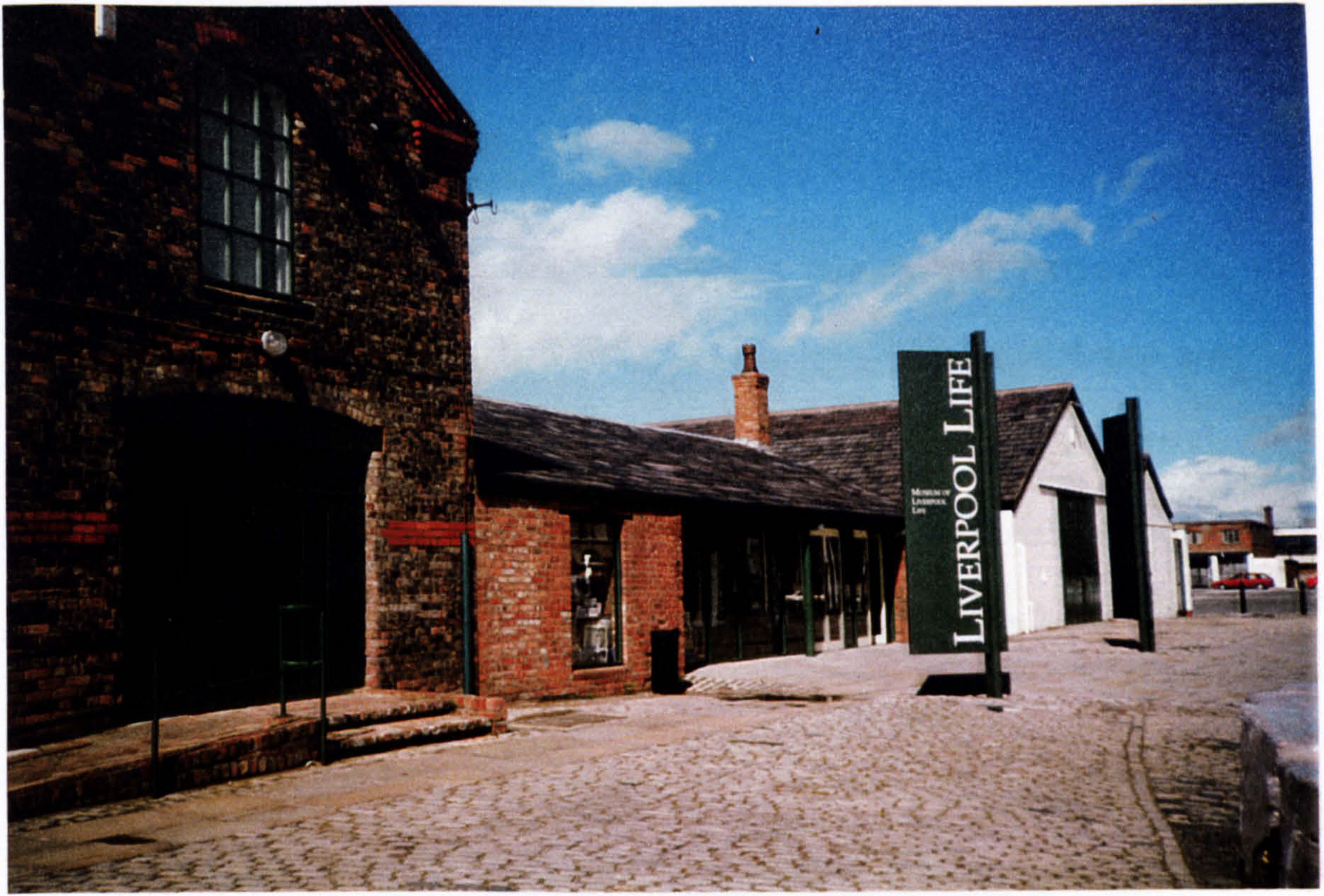
Photograph 3.1: The Museum of Liverpool Life, Albert Dock, Liverpool
