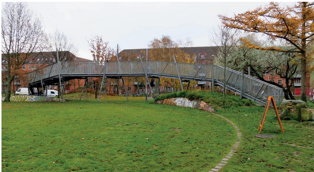
Fig. 11 – Folkets Park before the renovation (Image taken by Kenneth A. Balfelt).
