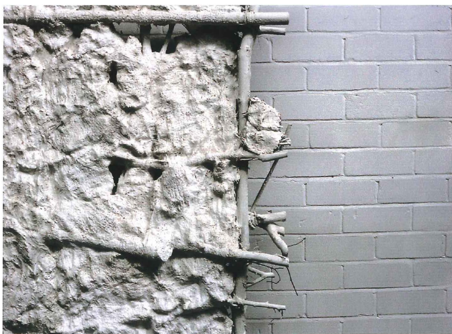
Fig.32 Panel III with studio brick wall
