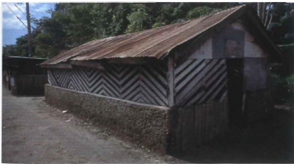
Fig.18 Local vernacular architecture - wood, cement, mbati , tin
