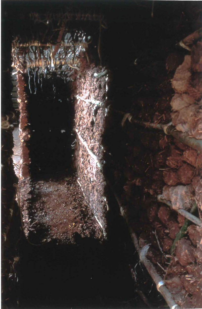
Panel cut away from side wall
