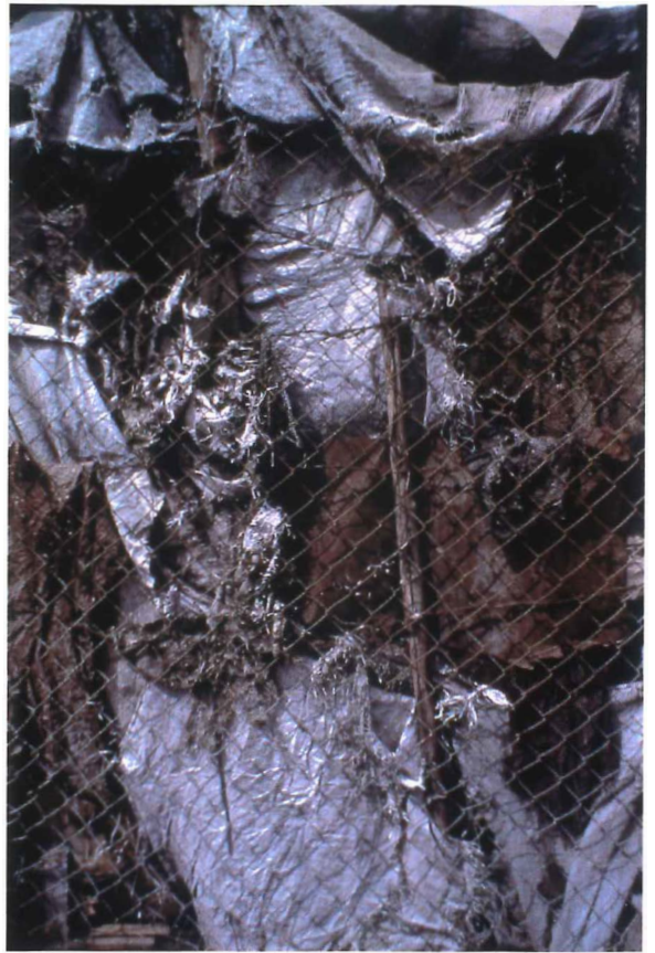
Fig.17 Fence made of flour sacks sewn together
