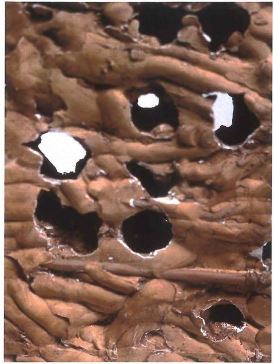
Fig.73 Wall with holes - detail
