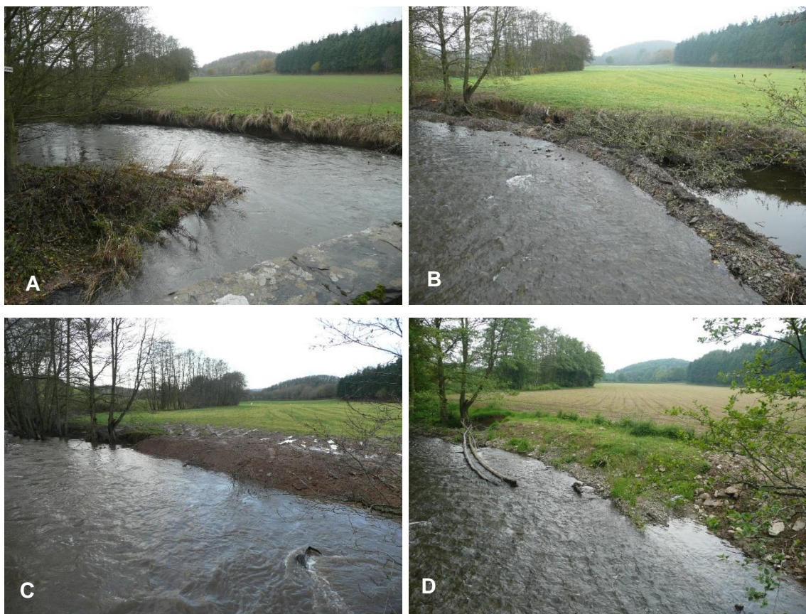
Figure 4.21 Bank protection scheme at Hunton Bridge, just upstream of monitoring site (a) evidence of bank erosion undermining bridge 18 th November 2009, (b) phase 1 base establishment 15 th November 2011, (c) phase 2 bank in-filling 13 th December 2011, (d) consolidated bank with erosion evident 4 th June 2012.
