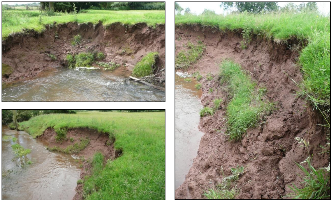
Figure 8.24 Examples of severe channel bank erosion and slumping in the mid and lower parts of the Cheaton Brook sub-catchment.
