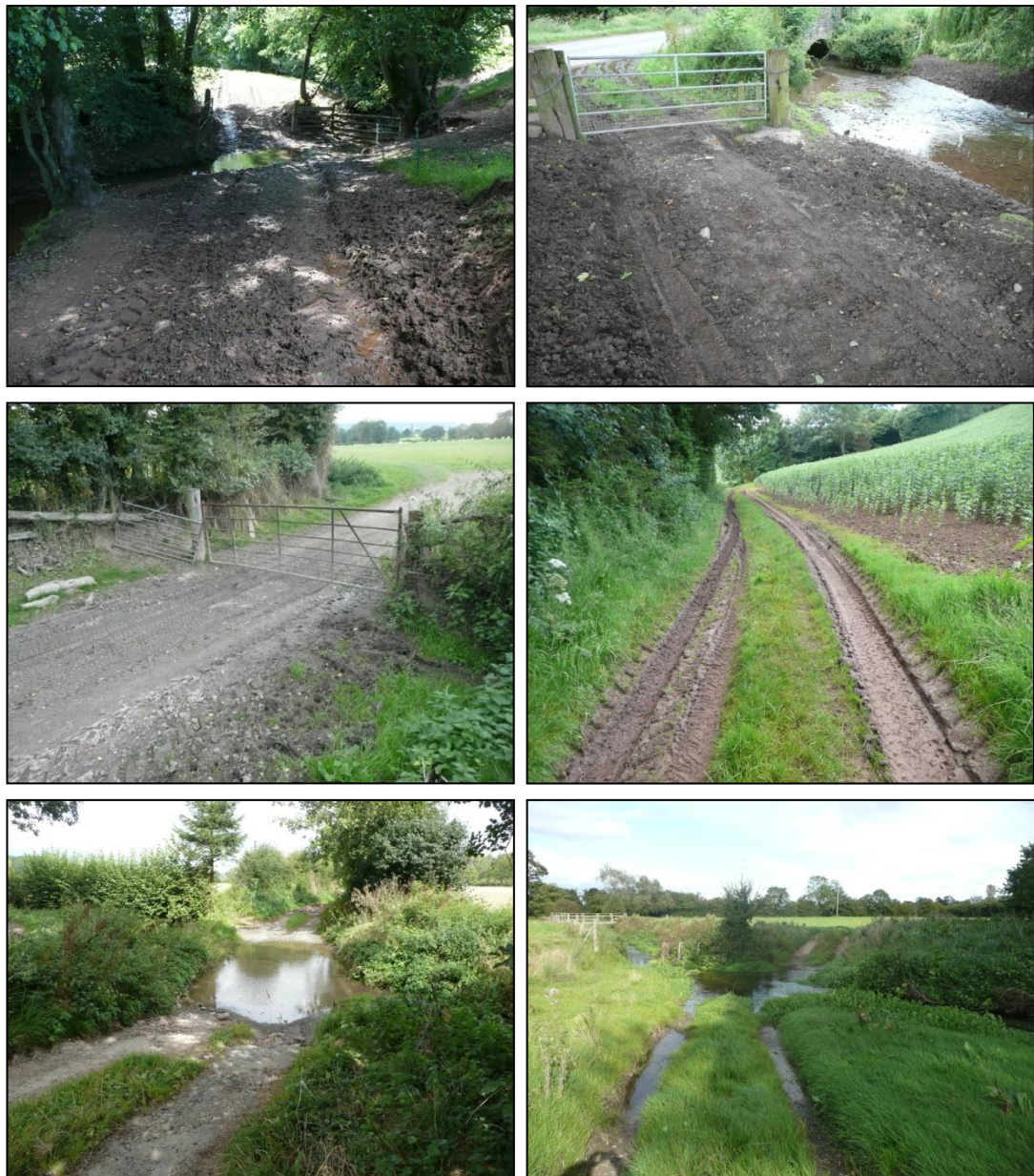
Figure 8.3 Typical characteristics of farm tracks located in the Cheaton Brook, Curl Brook and Moor Brook sub-catchments, demonstrating greater connectivity with the channel network and extensive surface damage.
