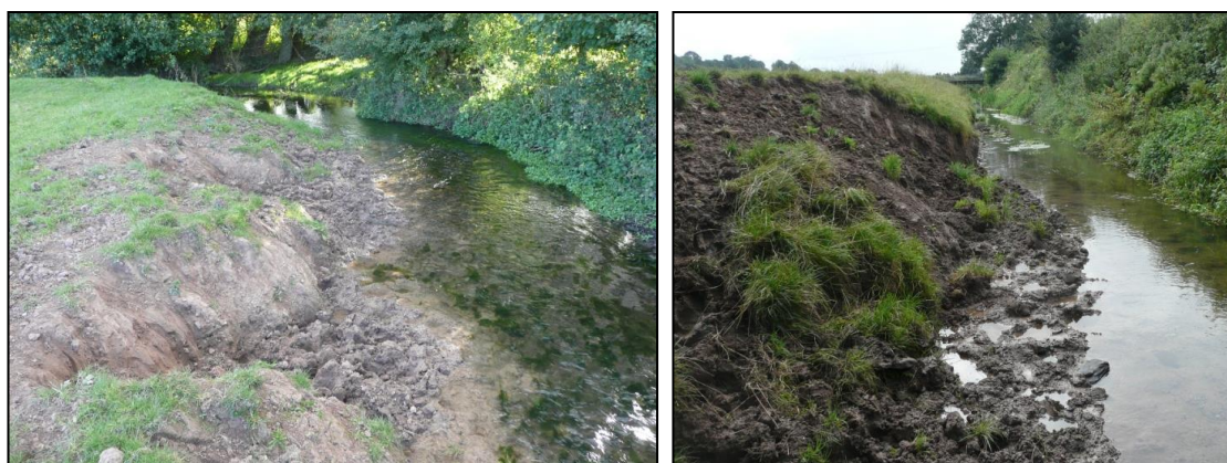
Figure 8.25 Examples of bank degradation and erosion in the Ridgemoor Brook and Curl Brook sub-catchments as a result of severe livestock trampling.
