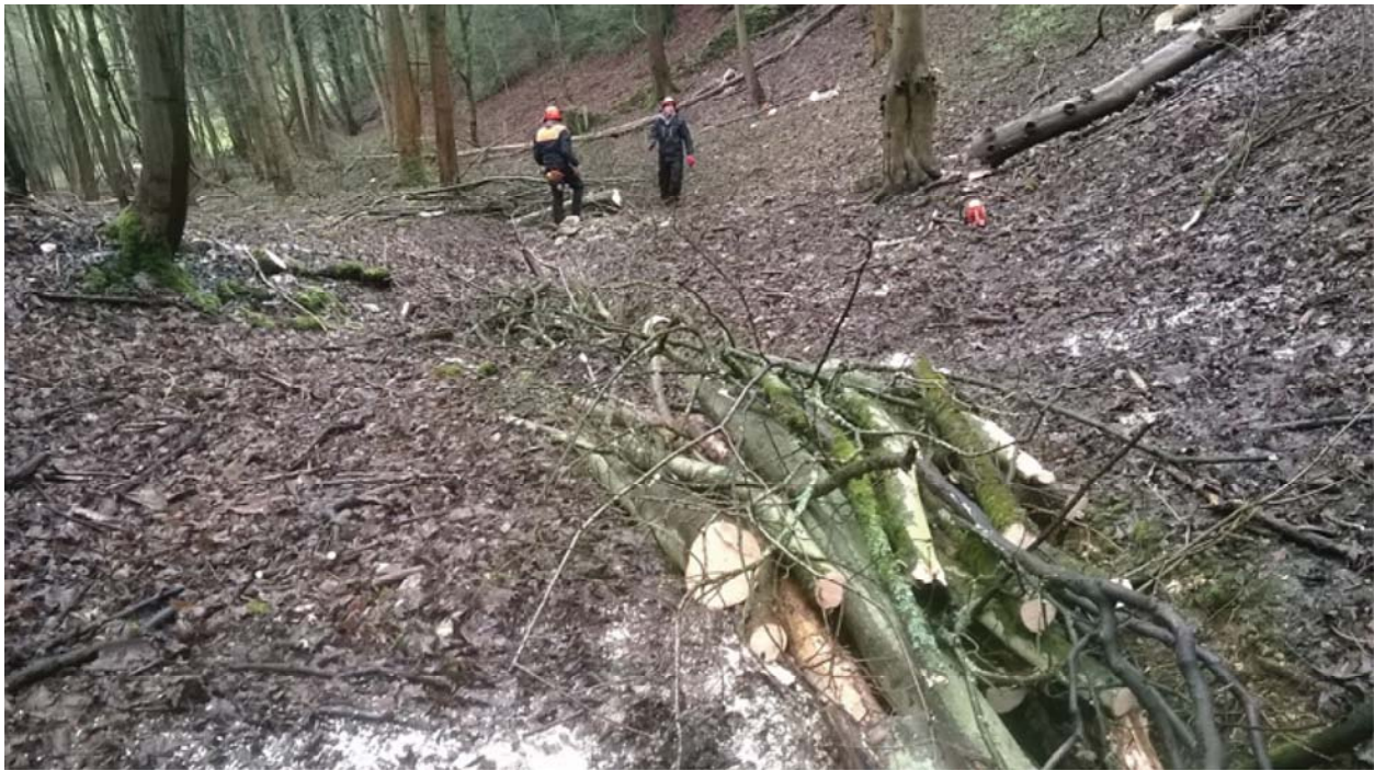
Figure 4: Example of gully stuffing in the Stroud Frome Catchment using brush and small logs to reduce surface runoff in the steep-sided valley
