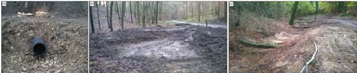
Figure 6: Examples of the culvert and grip interventions that have been implemented in the Stroud Frome Catchment to reduce surface runoff and material transportation from tracks (a) large culvert pipe and stone soak away in a catch pit under the inlet pipe, (b) a track-side storage area (c) grip created alongside tracks
