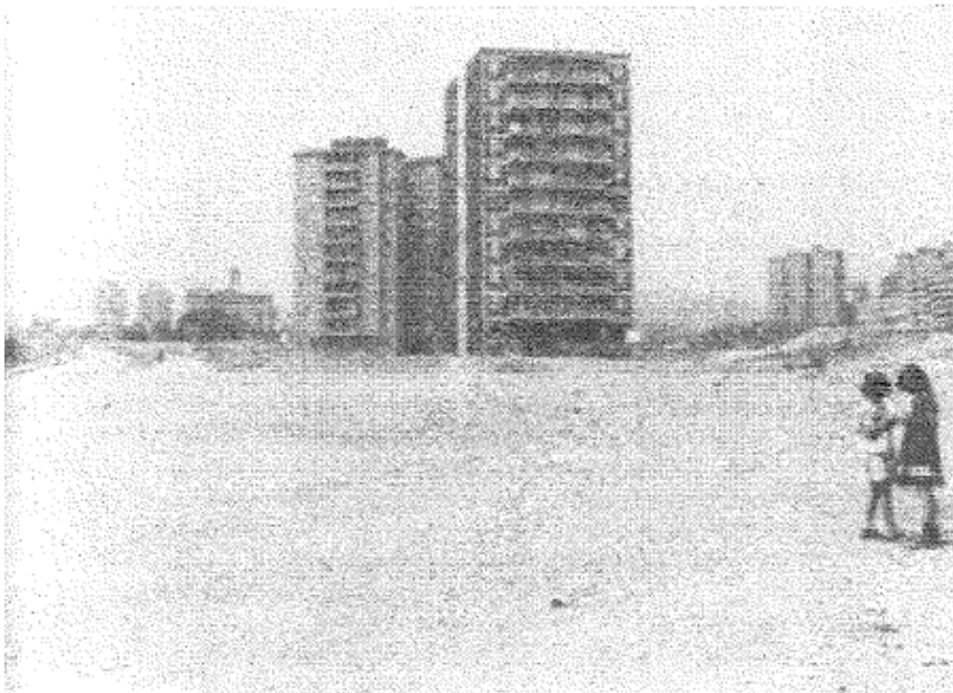
Figure 5.12 Can Serra, Hospitalet, Barcelona. Lack of local authority finances have often prevented the provision of service infrastructure contained in Local Plans for housing areas. Here, children play in an area in which a sports centre, public gardens, health centre and school should have been built. Photo: M.G. Wynn.
