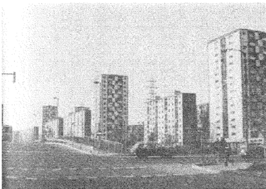
Figure 5.7 The ‘La Paz’ Housing Estate (2,499 houses) in the Municipality of Barcelona. This estate was built between 1963 and 1966 by the Syndical Housing Authority (OSH) at an average density of 591 inhabitants per hectare. Photo: M.G. Wynn.
