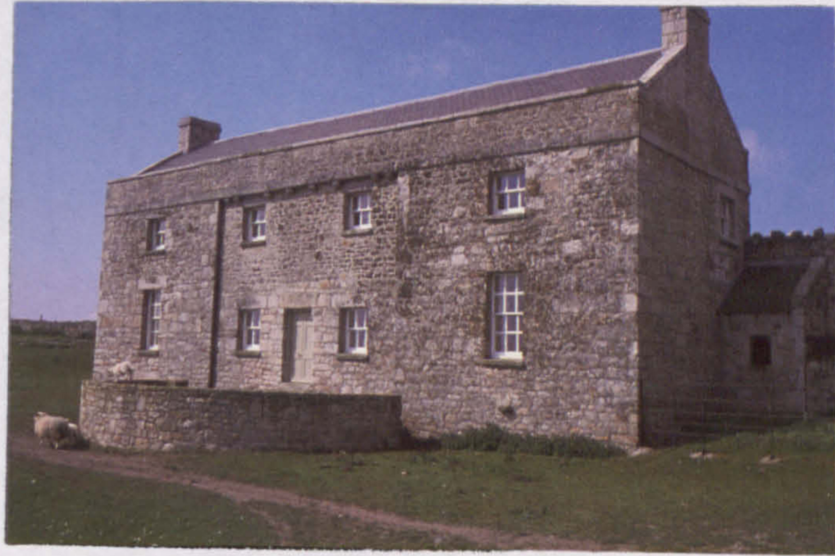
EAST FACADE, PRESENT OLD HOUSE
