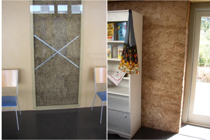
Figure 3.4.2: Exposing straw bale and rammed earth materials in the Genesis Project at the Somerset College of Arts and Technology
