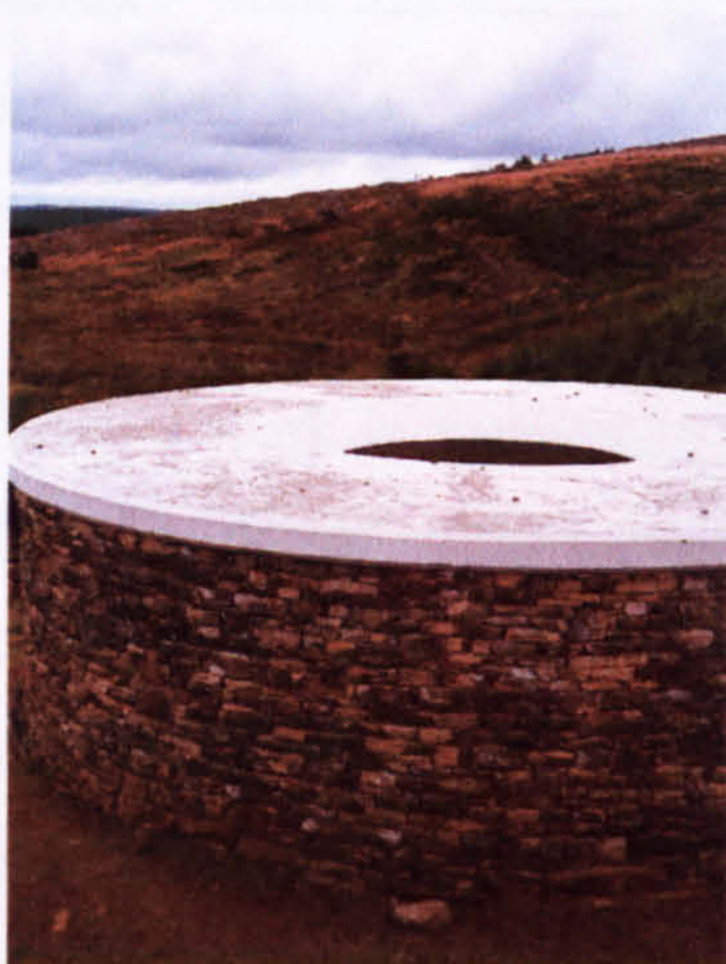
Fig. 55 Skyspace , 2000 (Roof) James Turrell Keilder
