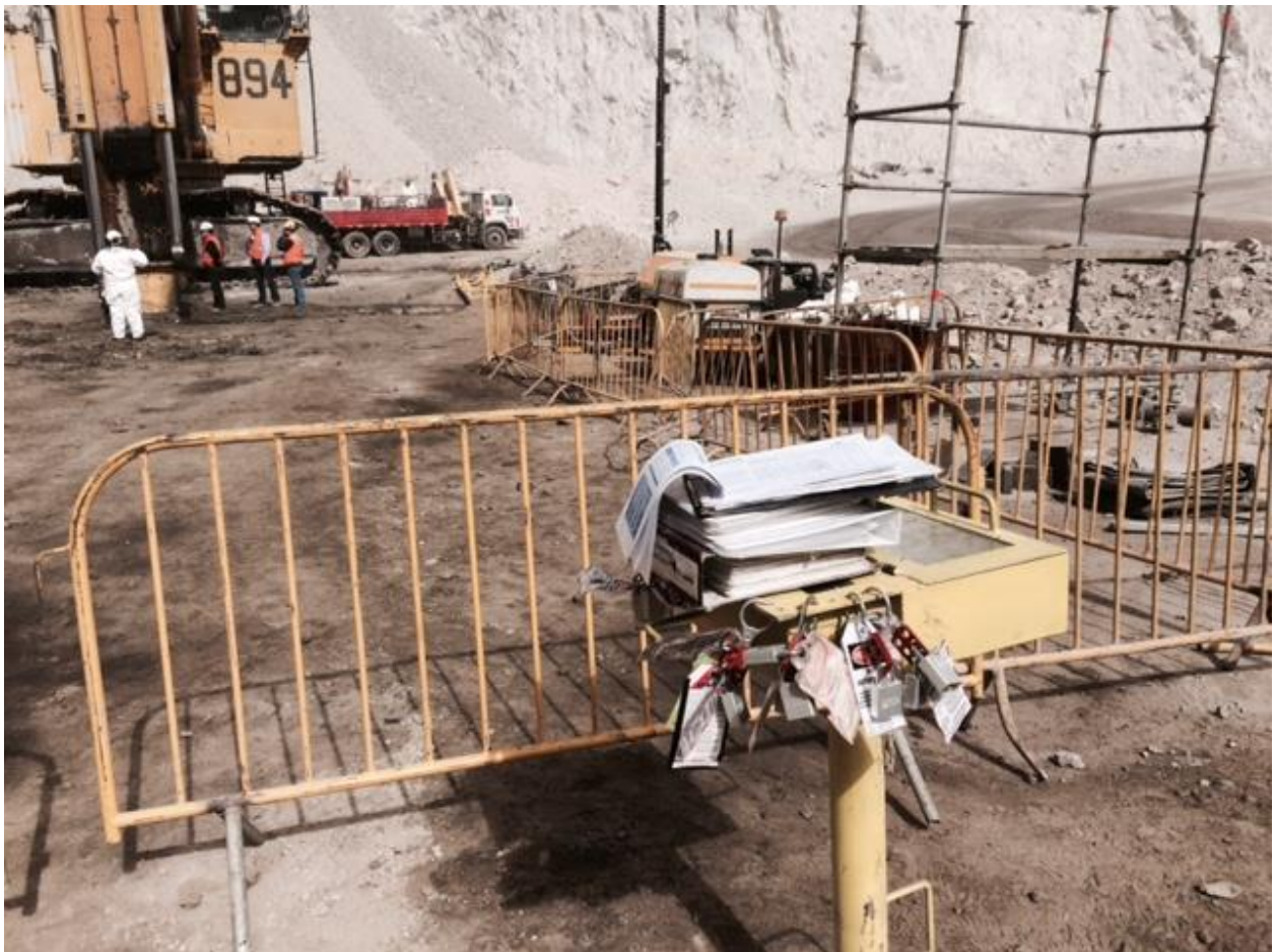
Picture 6: The locking station in front of the fence that delimits the working area.
