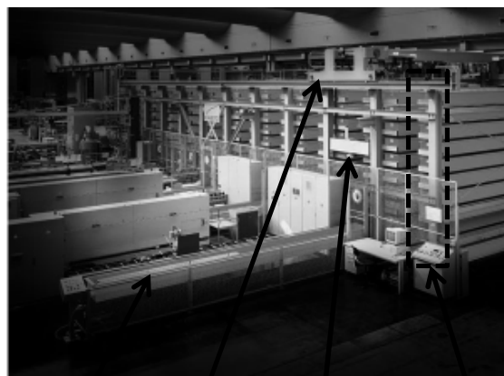
Transfer station / rails crane / removal traverse / cantilever rack
