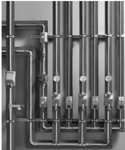
Figure 1.2: Installed Pipes (Viega GmbH & Co. KG, 2014, p. 14)
