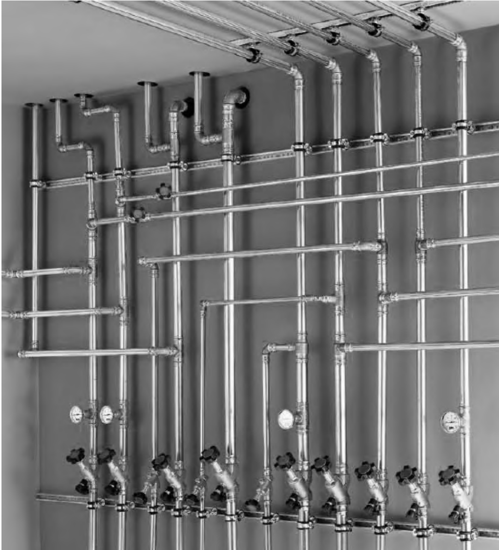
Figure 2.5: Water Pipes (Viega GmbH & Co. KG, 2014, p. 8)
